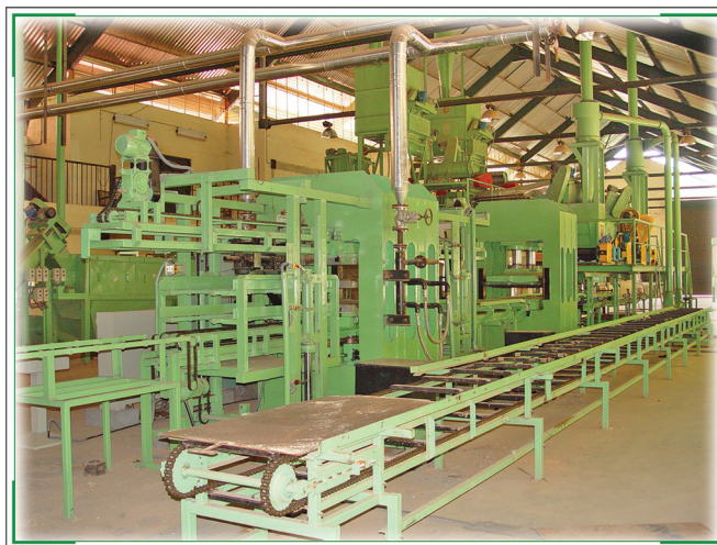
PARTICLE BOARD PLANT
