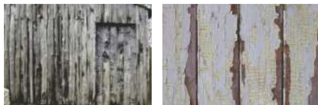
Fig. 1 Weathered wood and coating failure
